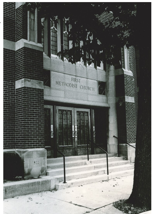
Cornerstone of the church dated 1922 as seen on the 7th street entrance. Picture taken in 1977.
